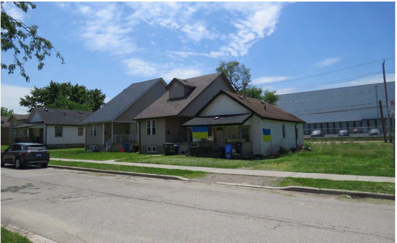
987 and 1003 California Ave (Subject Land) looking south west
